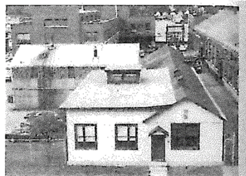
Electrical Certification Laboratory (554 Booth St.) 1954, on site of old machine shop; new machine shop (556 Booth St.) is at left rear; Butler building for carbonization studies is in middle rear
